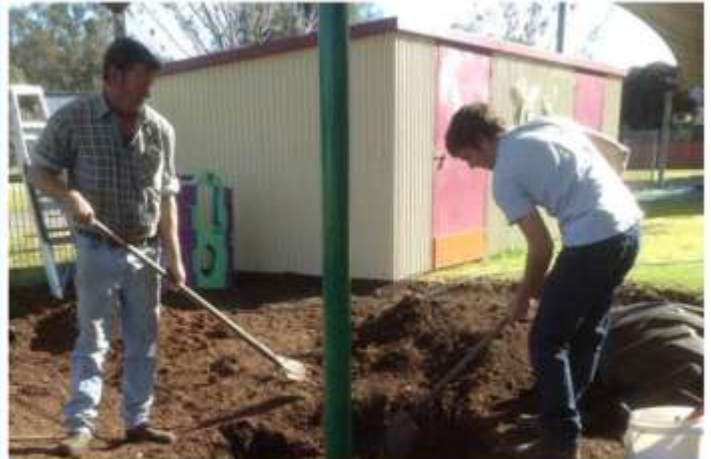
Lance and Luke putting in the new equipment
